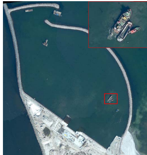
Figure 7: Harbour construction, 14.4.2004, 16 cm GSD, mosaik of 12 images, covered with PFIFF
